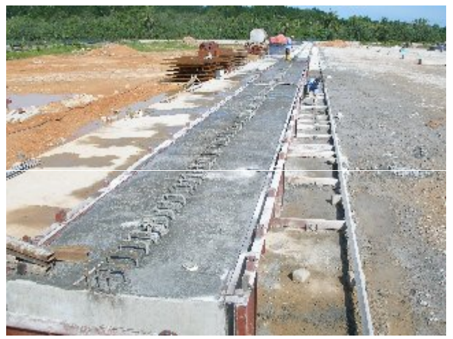
Single Tee Beam Mould
