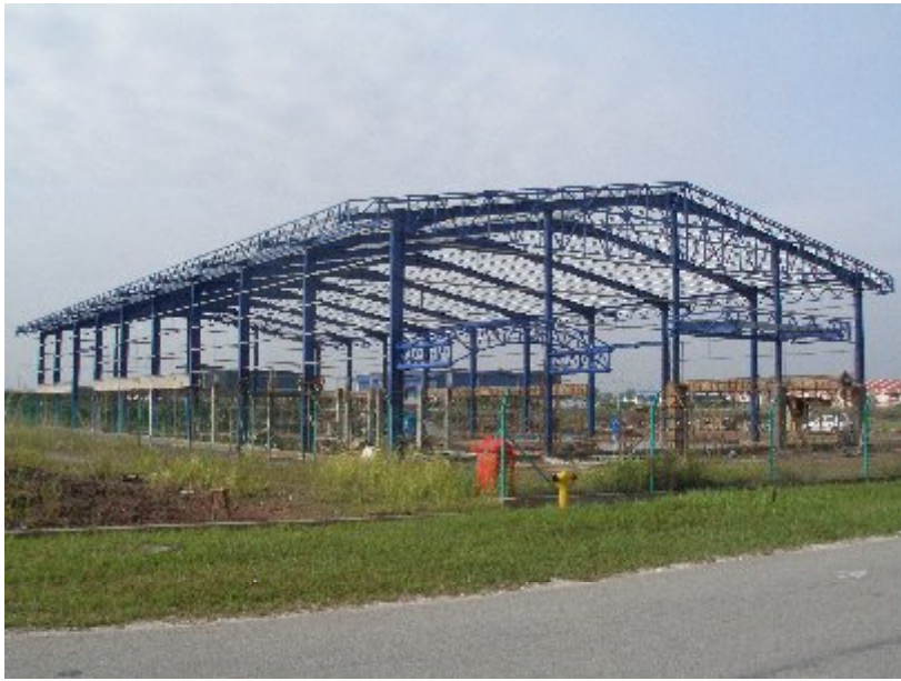
Factory Structure Steel Fabrications
